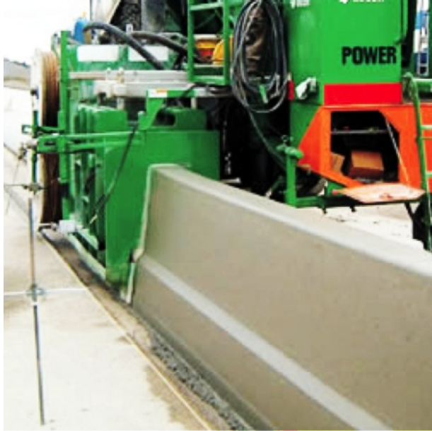
Left: A slip form paver lays a continuous concrete barrier. (Photo credit: Powercurbers ) Right: A toy pushes clay in a similar (though far more simple) way. (Photo credit: Wikipedia )
