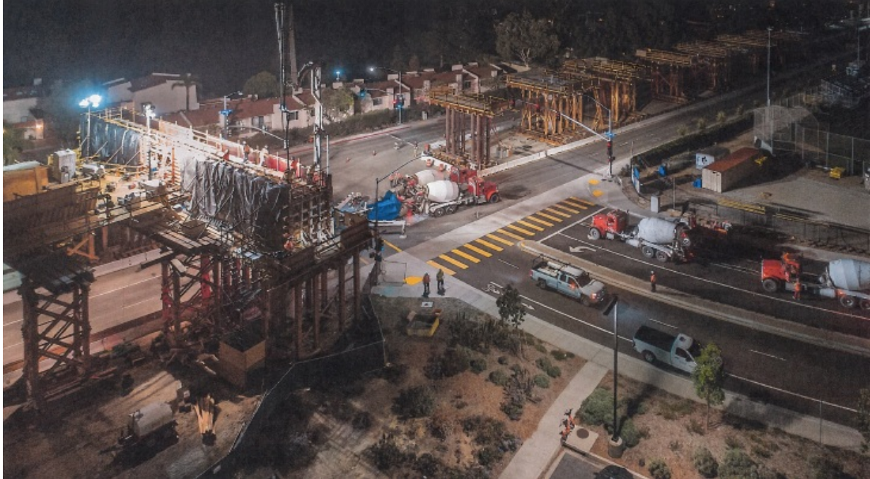
Concrete trucks staging, about to begin the outrigger pour.
