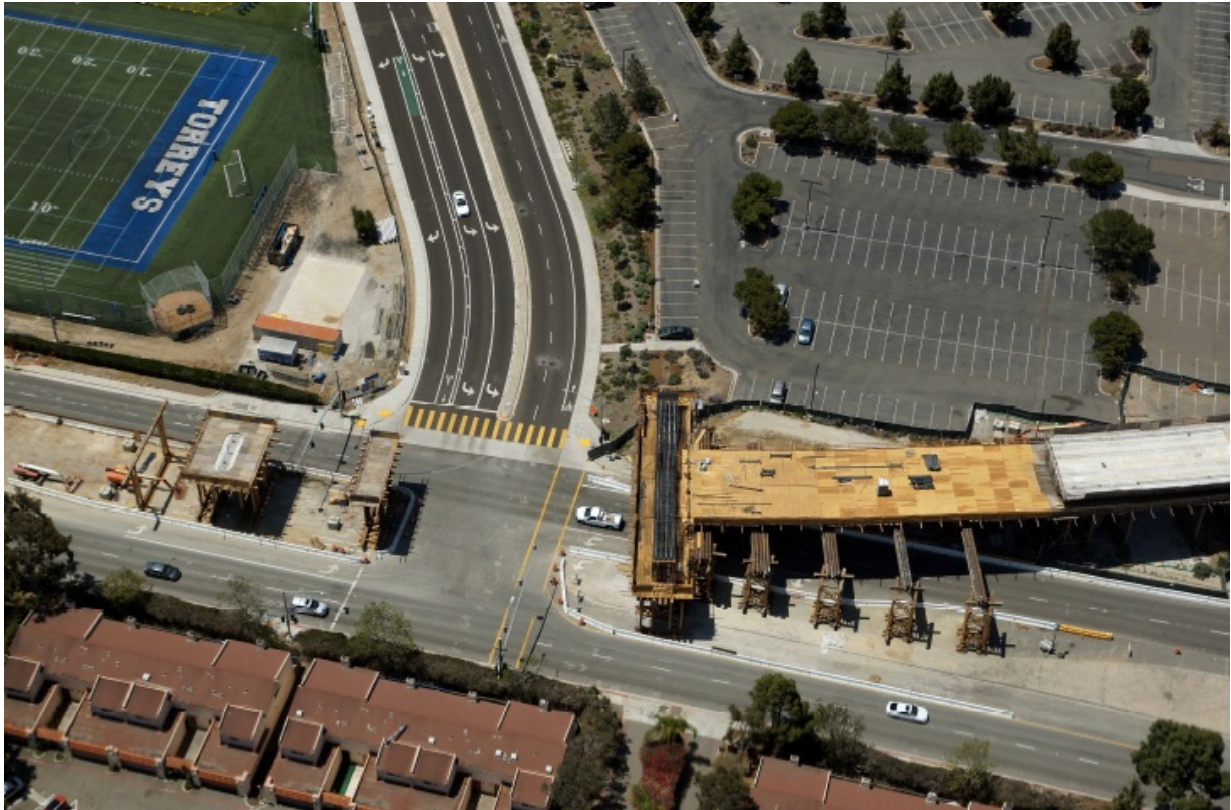
Aerial view of Genesee Viaduct. Outriggers can be seen in lower right corner.
