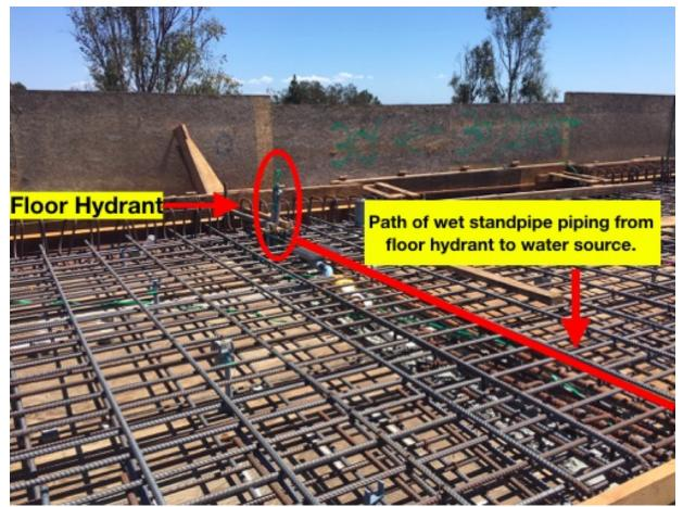
Future Voigt Station on the Mid-Coast Corridor Transit Project: In preparation for a deck concrete pour, the wet standpipe piping is installed prior to the rebar.
