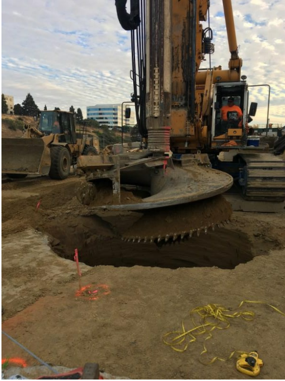
Installing a CIDH foundation for a Viaduct on the Mid-Coast Corridor Transit Project: On the left, a drill rig digs a 120 foot deep shaft. On the right, workers prepare the rebar cage for installation into the drilled shaft.
