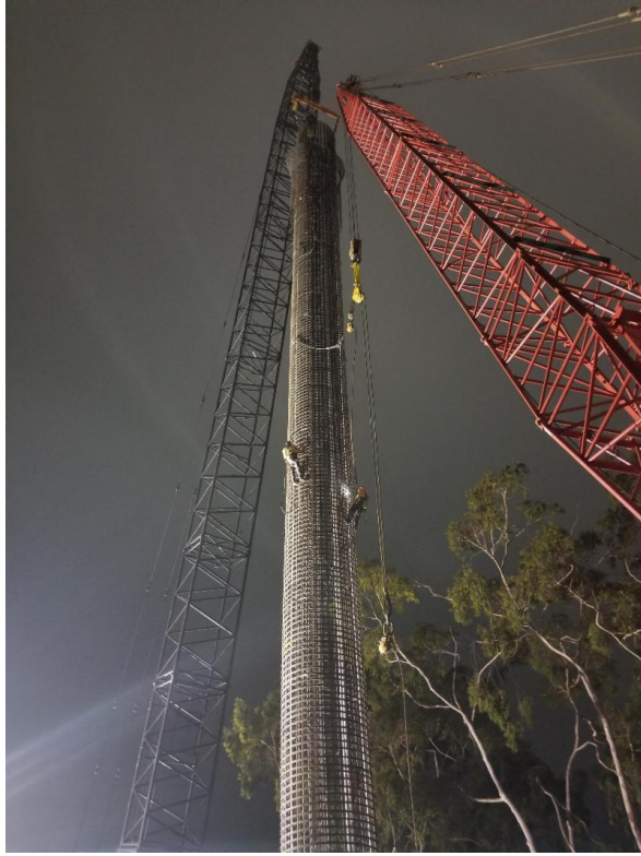
156' crane being lowered into a drilled shaft.
