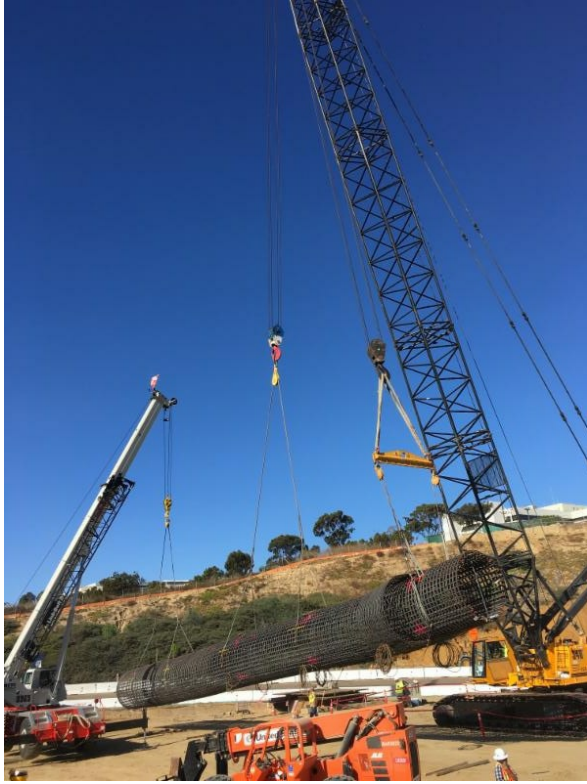
Rebar cage being hoisted by 2 cranes.
