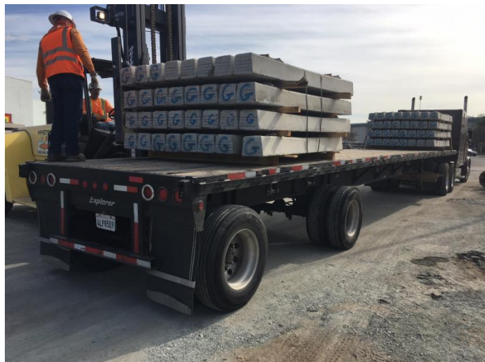
MCTC unloading concrete ties from a flatbed truck.
