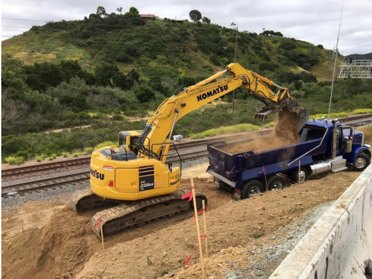
Dump truck being loaded with wall excavation spoils.
