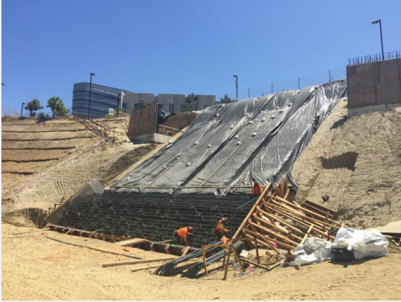
Gilman Bridge abutment
