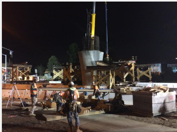
Frame 15 falsework over Campus Point Drive
