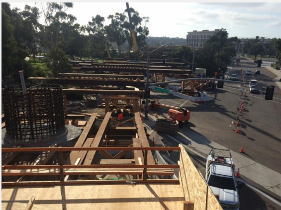
Falsework installation at Campus Point Drive
