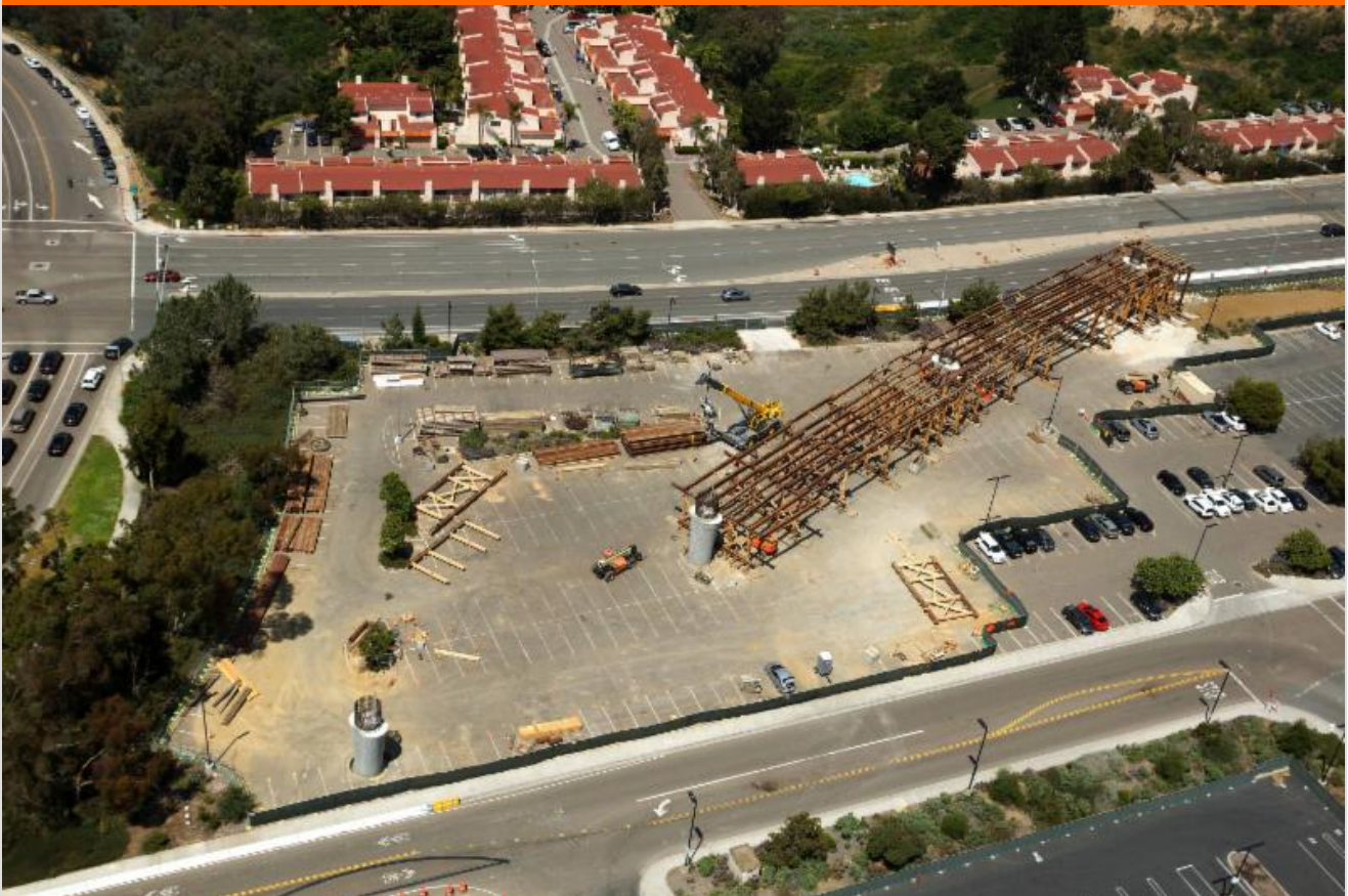
UCSD Viaduct falsework installation near Campus Point
