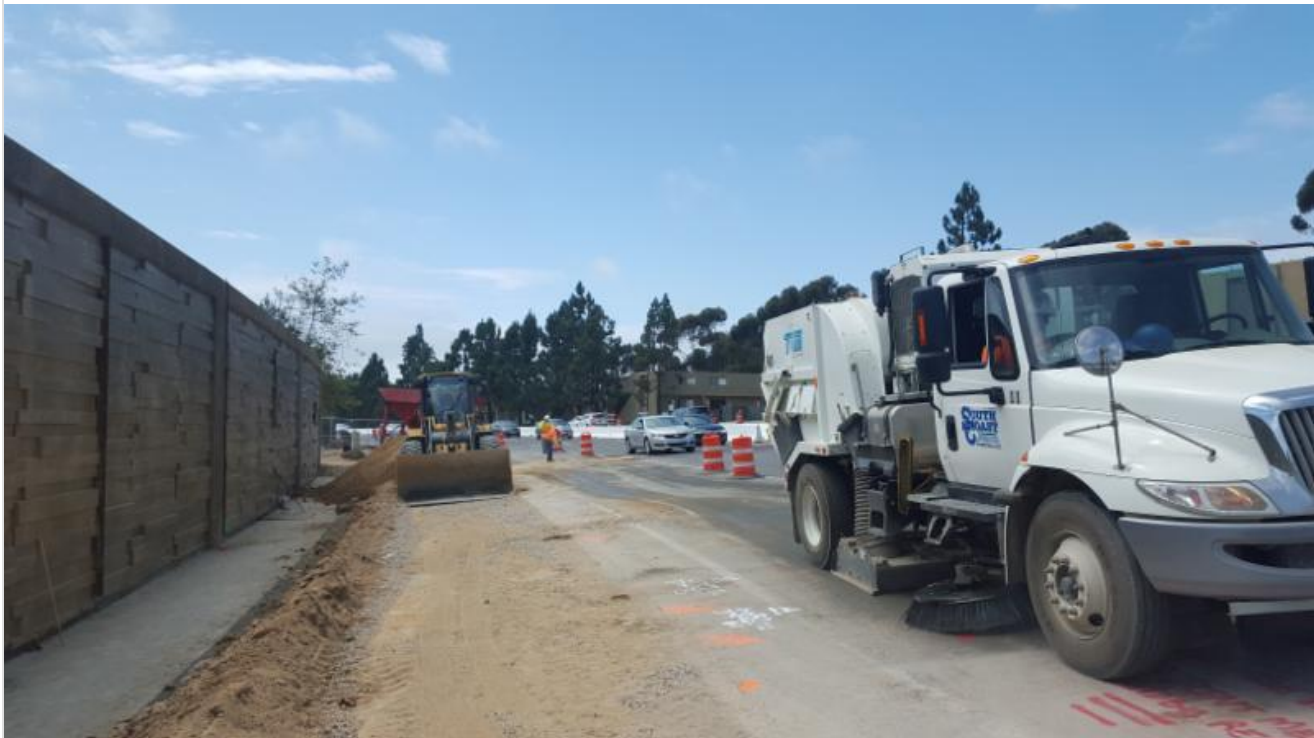
Genesee retaining wall almost completed
