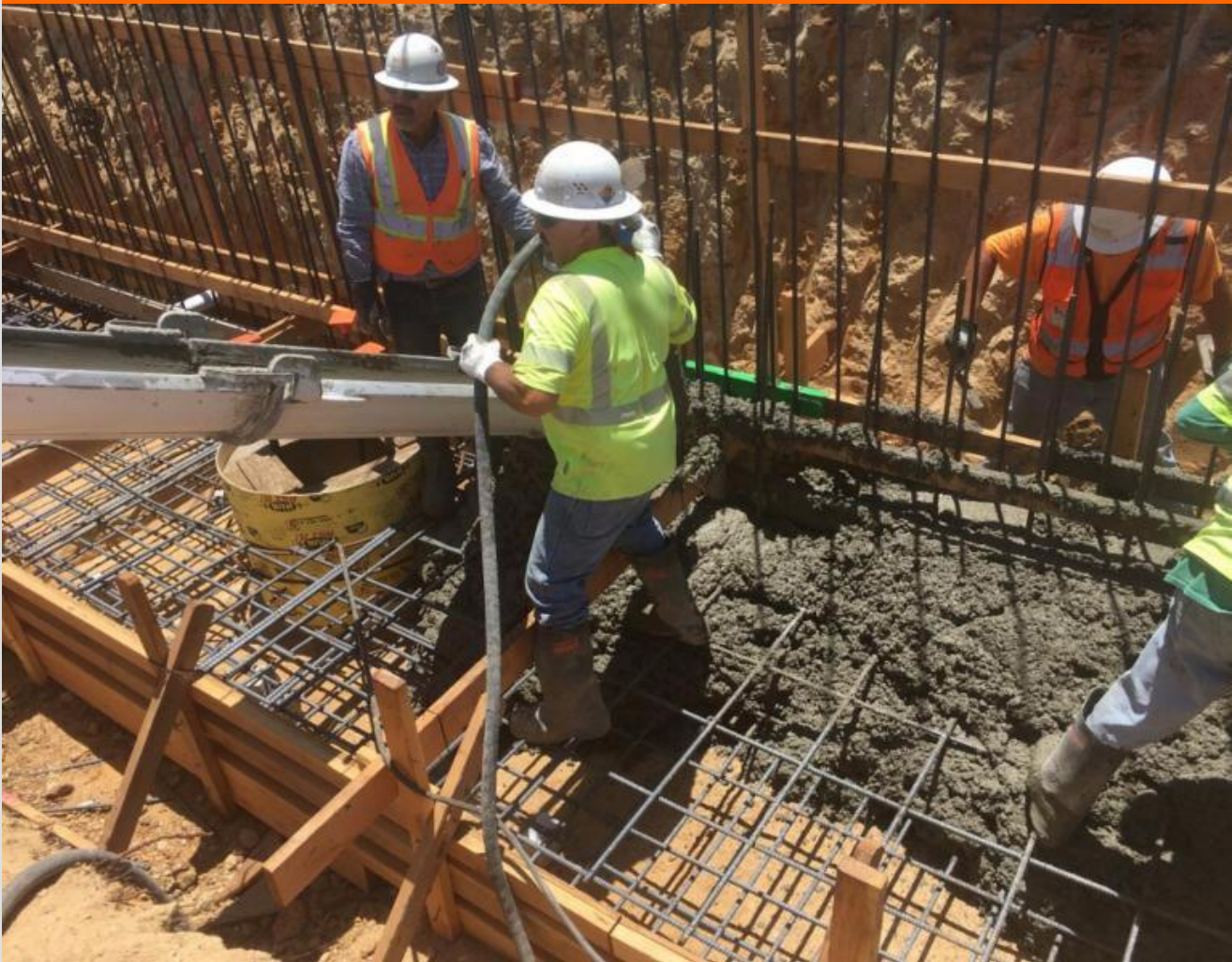
Early stages of retaining wall on Genesee
