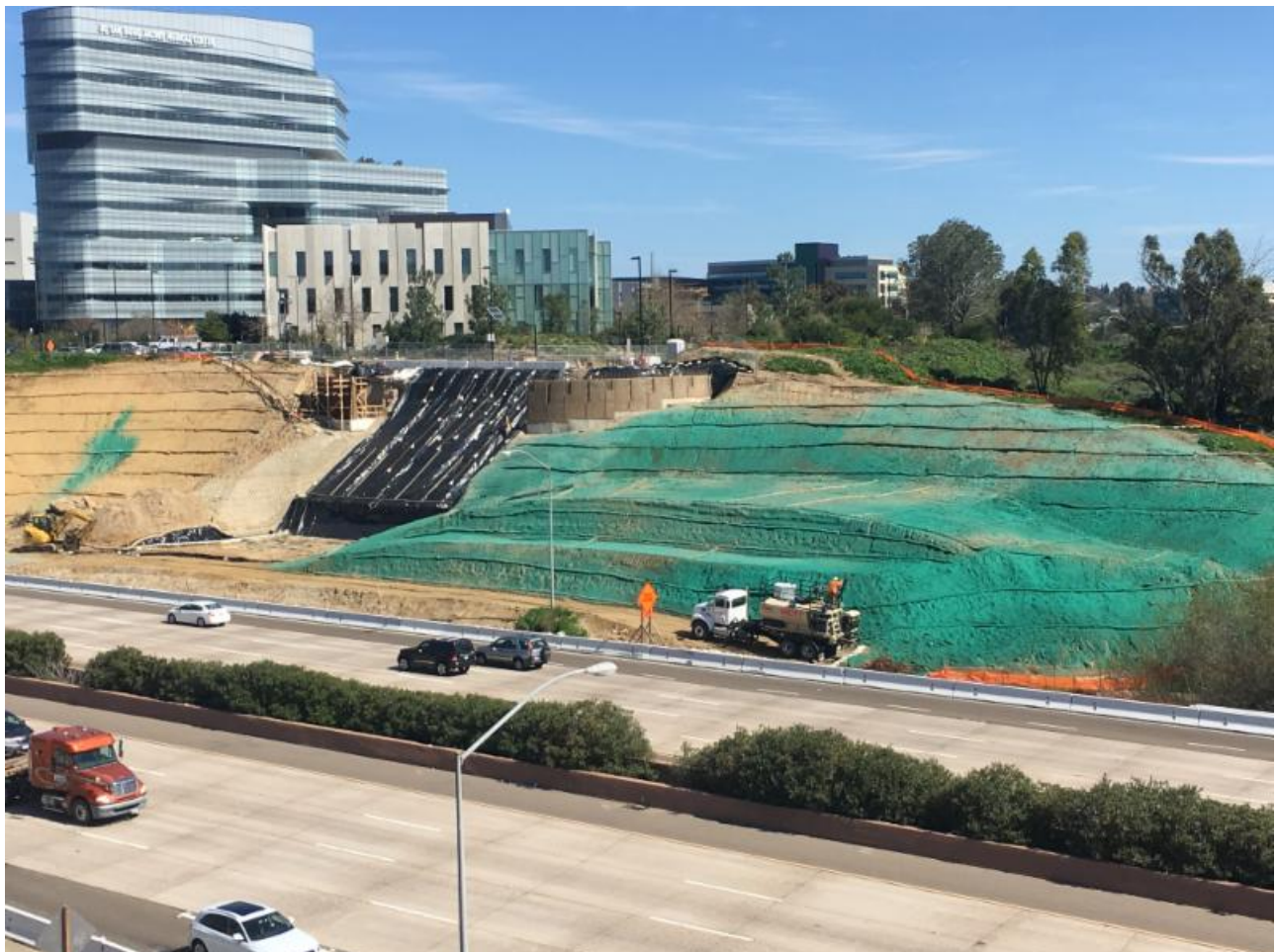
Gilman Bridge abutment construction on the east-side of Interstate 5
