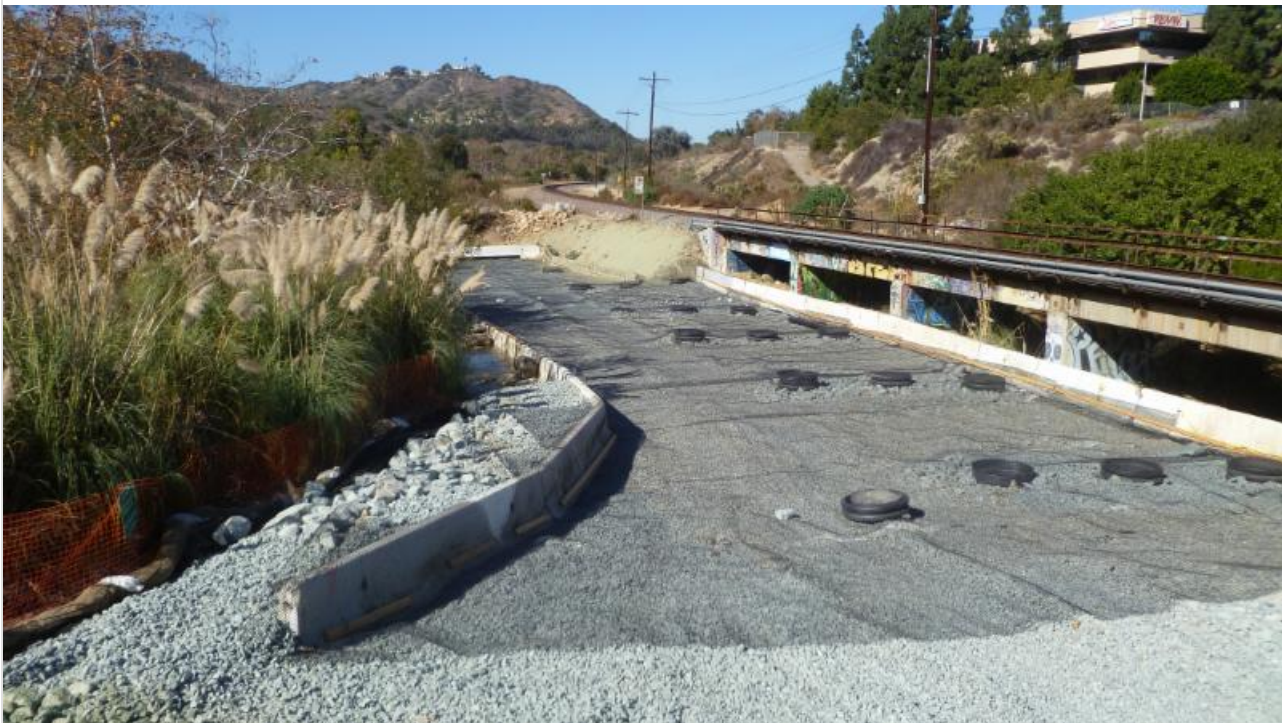
Bridge 259.1 all-weather access road built for bridge CIDH drilling
