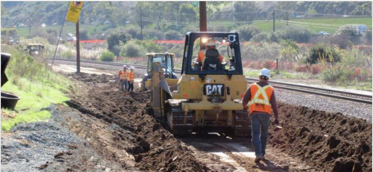
Access road excavation and grading
